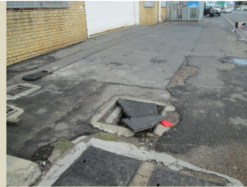
Figure 19 Broken manhole covers on sidewalks
