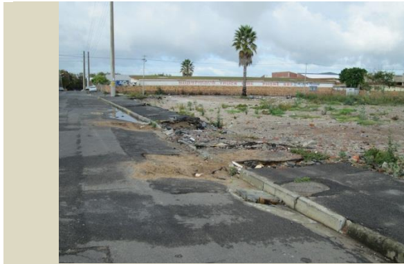
Figure 18 Unmaintained sidewalk surfaces
